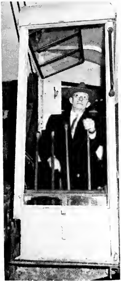
Governor Lane operates earth moving equipment to start one of the new projects.
